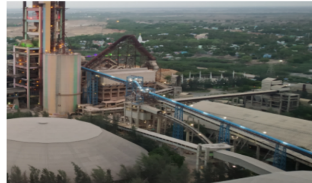
3. Conveying Belts 315 m
