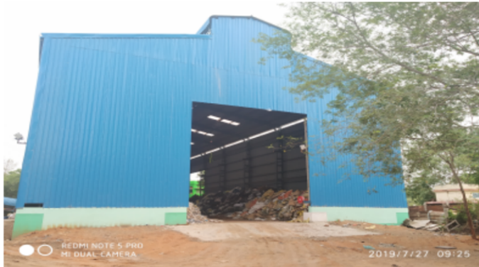
1. Shredded material Storage Shed
